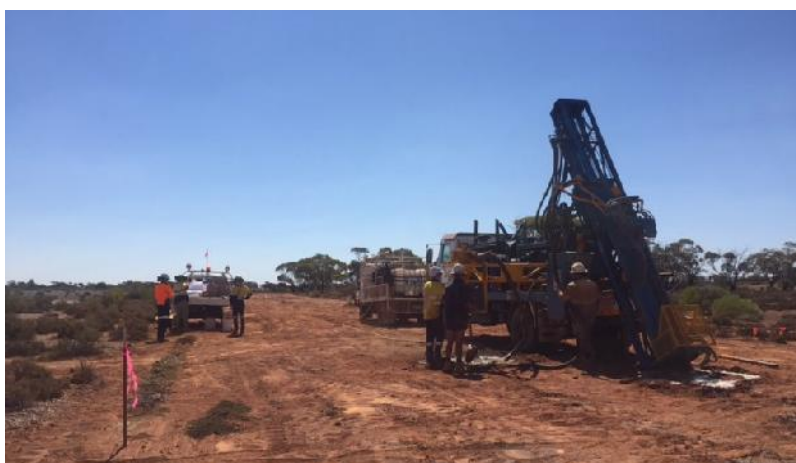
Figure 1 Aircore drilling underway at the Atlanta South Prospect – 30 January 2019.
